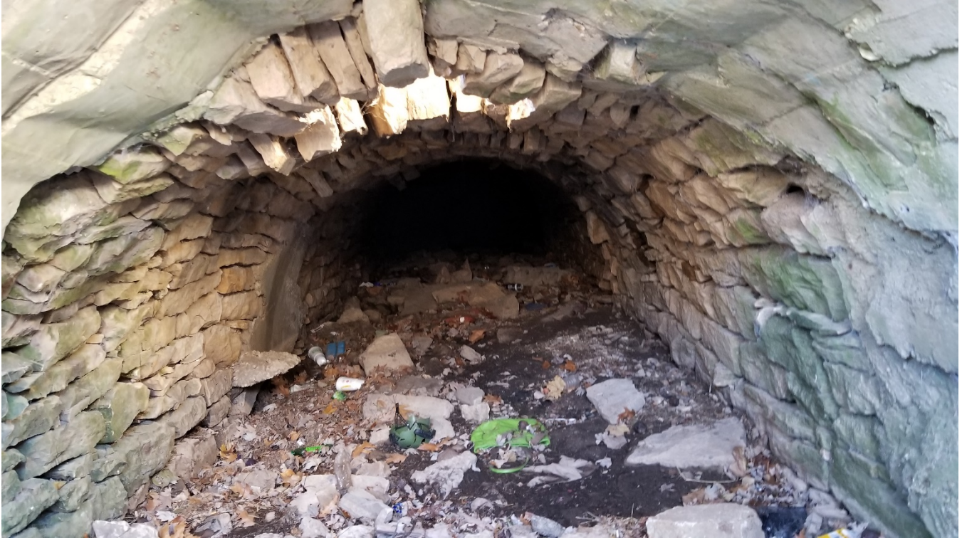
STONE ARCH STORMSEWER, LOOKING WEST FROM FULTON AVE
