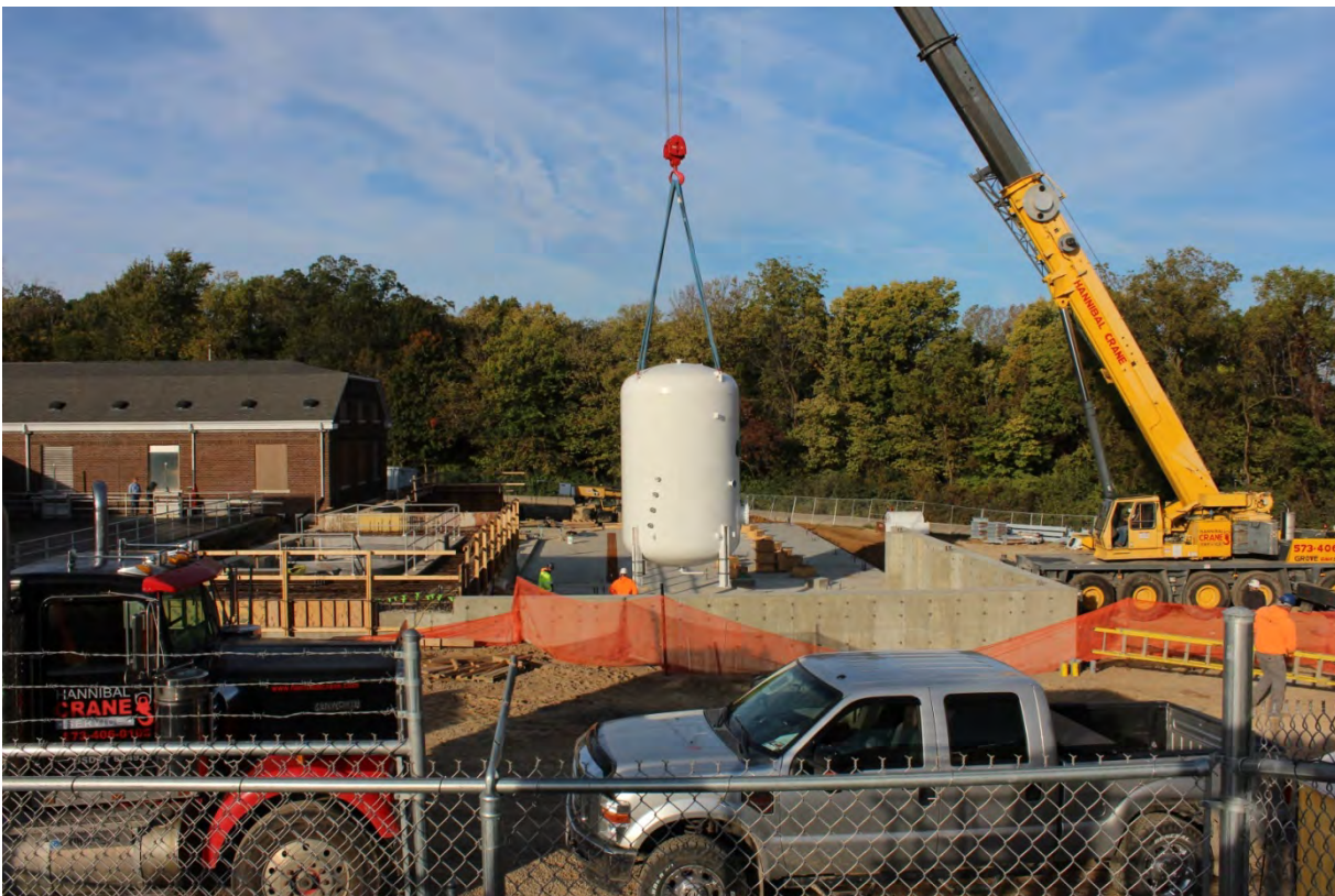
Figure 8: Setting of the first GAC vessel on October 18, 2019.
