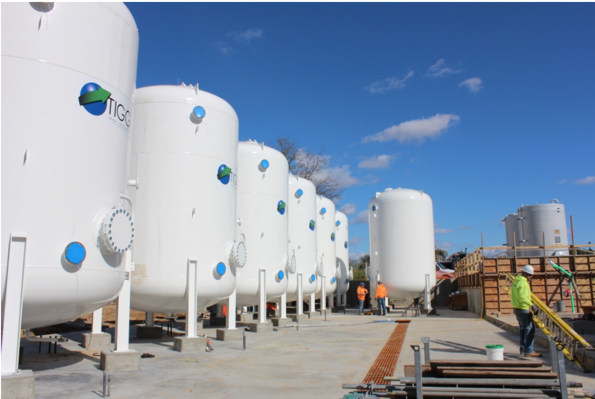
Figure 9: Picture after the eighth GAC vessel was set into place on the afternoon of October 22, 2019.
