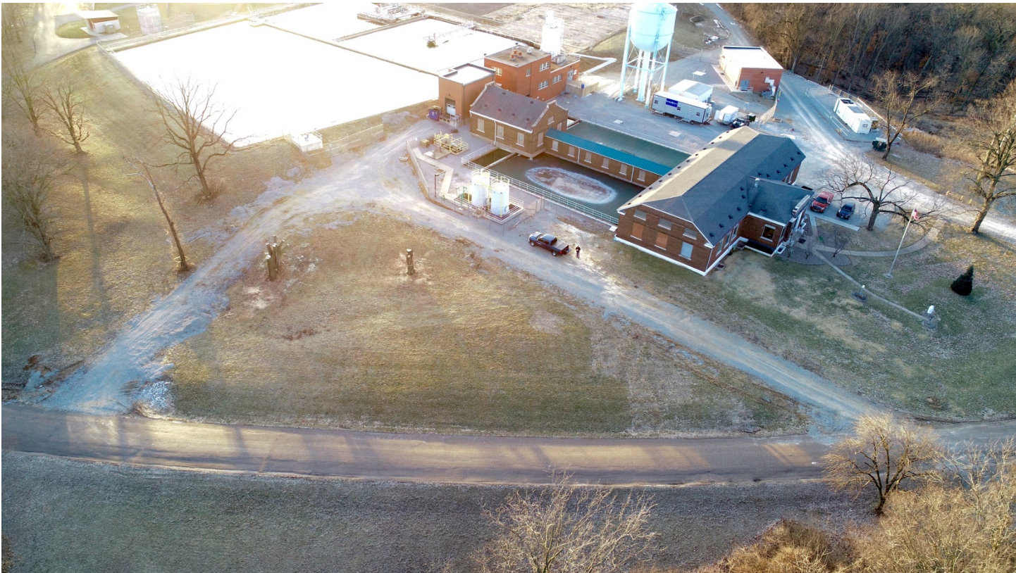
Figure 1: Photo looking from the north towards the project site taken in late February.
