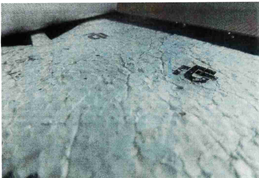
Figure 86: Dented substrate.
