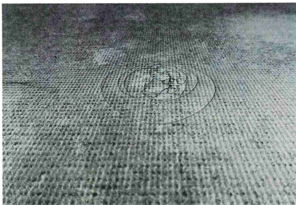
Figure 82: Hail damage to the PVC.
