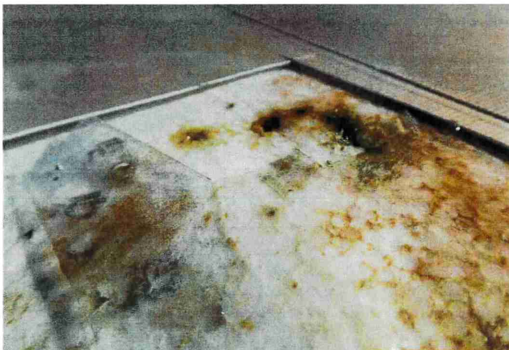
Figure 88: Water intrusion into the substrate.
