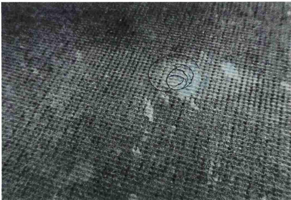
Figure 80: Hail damage to the PVC.
