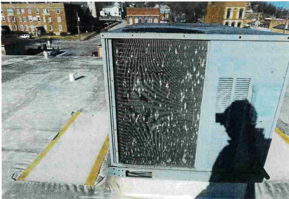
Figure 77: Dented air conditioning fins on City Hall.
