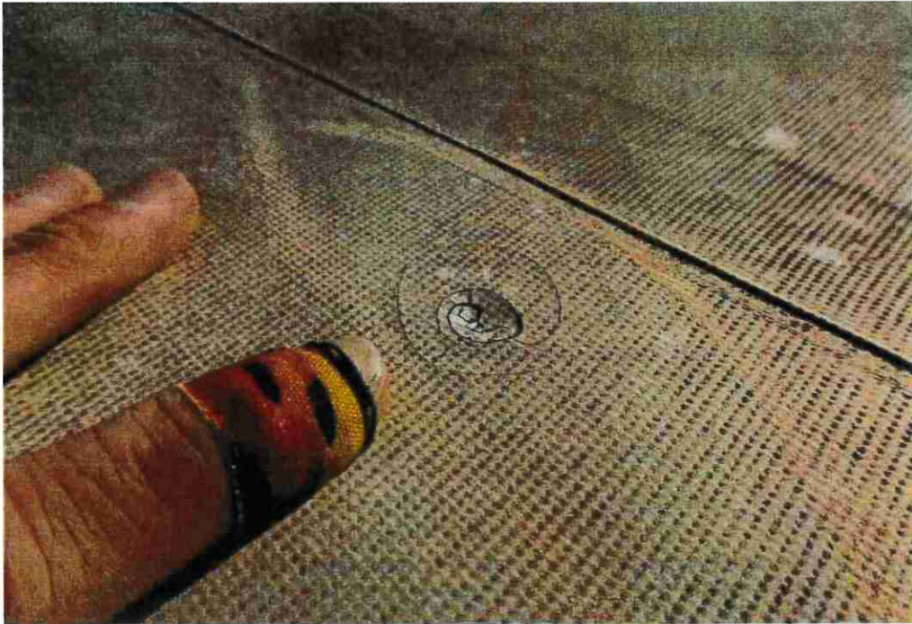
Figure 79: Hail damage to the PVC.
