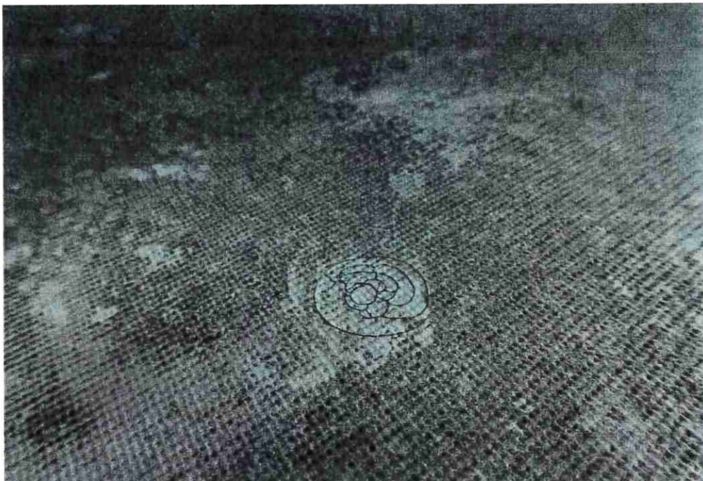
Figure 81: Hail damage to the PVC.
