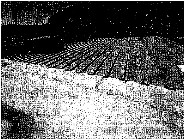
STRUCTURAL METAL ROOF PANEL SYSTEM PHOTO 5
